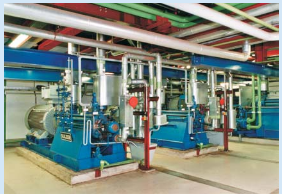
MC 80-260, 13 stages, Head 1360 m, Capacity 100 m 3 /h, 517 kW
